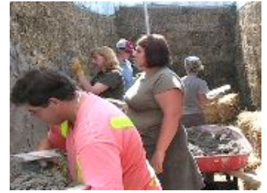
workshop wall plastering (from video)
