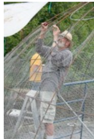
Jerrard attaching wire to dome structure
