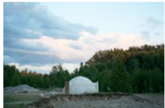
The ferro cement dome
