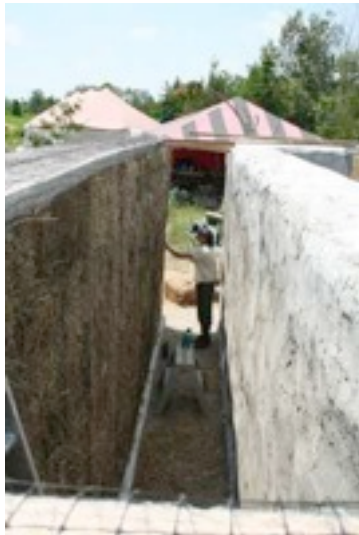
Walls ready to mortar
