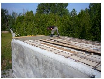
intensive workday. After some final reinforcement of the cement forms, mixing began. Two cement mixers were running continuously with one person operating each mixer. The mixed cement was poured into a plastic lined trough, from which another person shoveled cement into buckets. Another worker pulled the filled buckets up to the top of
