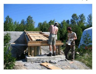
4x4s and plywood. For added strength, a rebar grid was laid inside the form before the concrete was poured. Aside from test mixes of concrete and the addition of cinder block supports under the ramp, the ramp construction took three full days.
