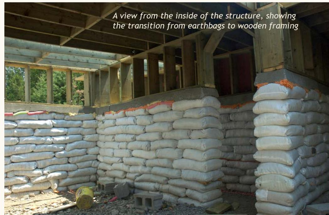
*A view from the inside of the structure, showing the transition from earthbags to wooden framing*
