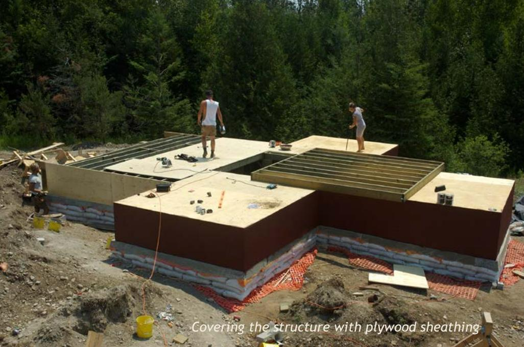
*Covering the structure with plywood sheathing*
