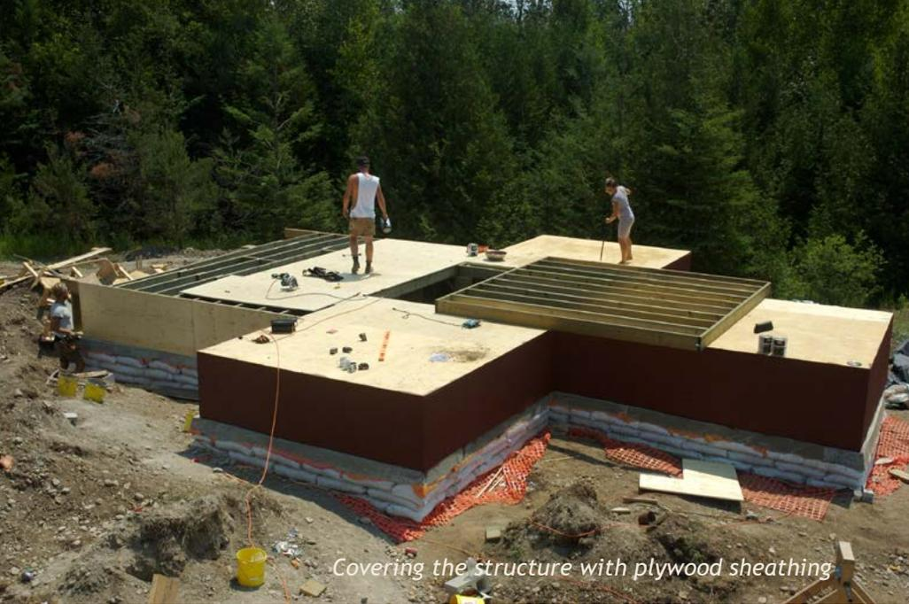
*Covering the structure with plywood sheathing*
