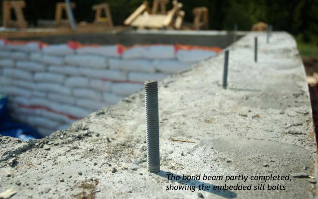
*The bond beam partly completed, showing the embedded sill bolts*
