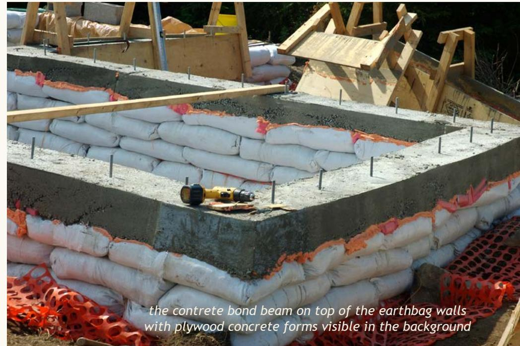
In order to build a sound wooden structure on top of the earthbags, a solid, level base was needed, so a concrete bond beam was poured on top of the earthbags, over which a PT lumber 2" x 10" sill board could be laid. Several 8' concrete forms were built using plywood and 2 x 4s. These were slightly flexible so that they could fit snugly overtop of the earthbag walls. The forms were re-used for all the walls as the crew moved around the perimeter pouring the beam. Plywood forms were then
